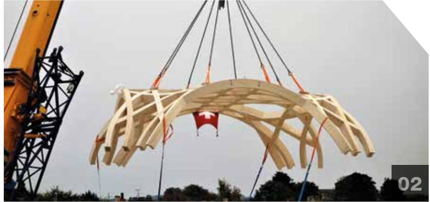
milled. The walls and ceilings were also prefabricated. Finally, these 600 elements and the 2,746 free-form pieces had to be lined up onsite. The high degree of prefabrication in the factory and thus the production under optimal conditions allows exact cost calculation, ensures high quality, super precise components and reduces the rate of error. Onsite, the advantages of prefabrication are made evident through short assembly time which has a positive impact on overall project costs.
